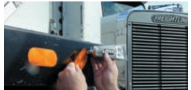
Install safety reflectors.
