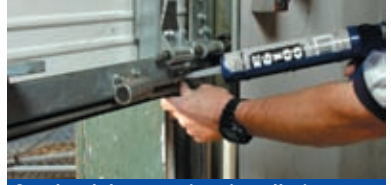
Overhead door repair & installation.
